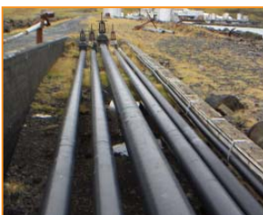
View from fuel jetty towards tank farm up on hillside
