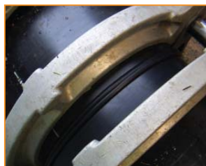
Close up of 315mm lined HDPE pipe in butt fusion machine
