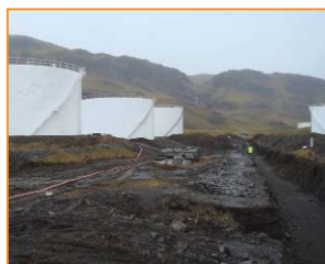
View of 4 of the 9 storage tanks in the tank farm
