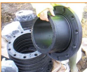
DN300 ANSI flanges and flange adapters used
