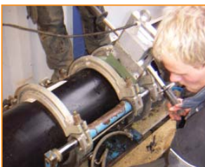
Pipe line constructed using butt fusion, saving on preparation time
